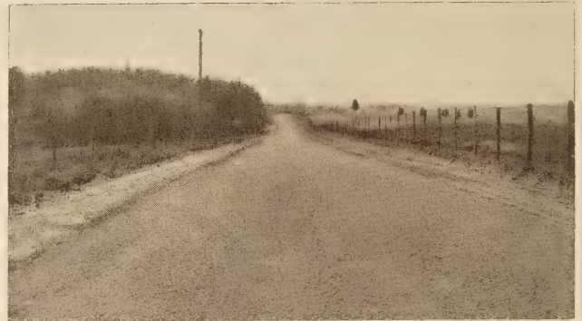
FIGURE 59.—SURFACE-TREATED ROAD OF GROUP A-2 MATERIAL IN MADISON COUNTY, VA.
